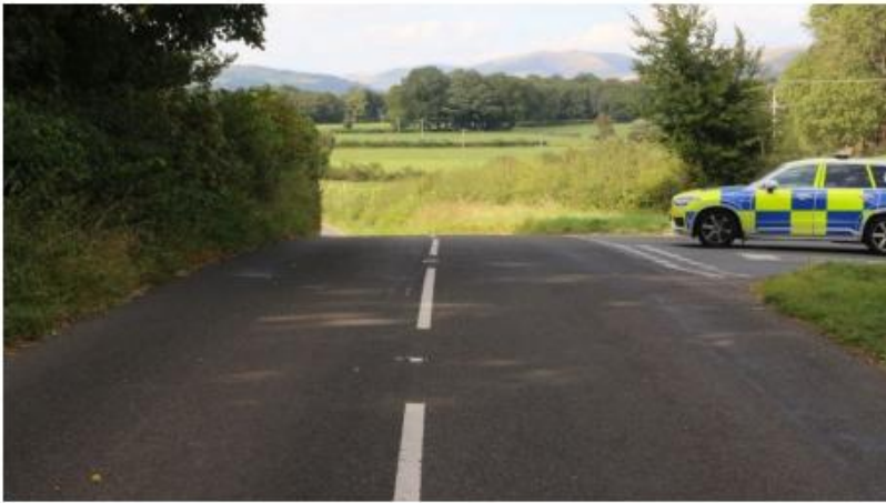
Figure 3 A scene photograph in the same position as Figure 2 but looking north in the direction of the collision scene. The blind crest next to the T-junction, in which a police car is parked. The subsequent bend in the A683 cannot be seen.
